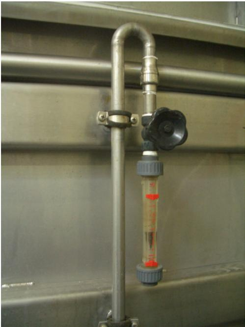
Air entrainment into suction pipe in front of inlet flange of DAF-pump
